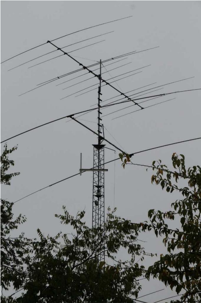
AREDN node k5ra-rk2o-parker77 is below the 2L full-size 40m beam and Force 12 C31-XR tribander antenna. The base of the node is about 75 feet up. There is also a TA-36 at about 50 feet. The tower is shunt-fed for 160m, and an 80m vertical will be re-attached soon below the AREDN node.
