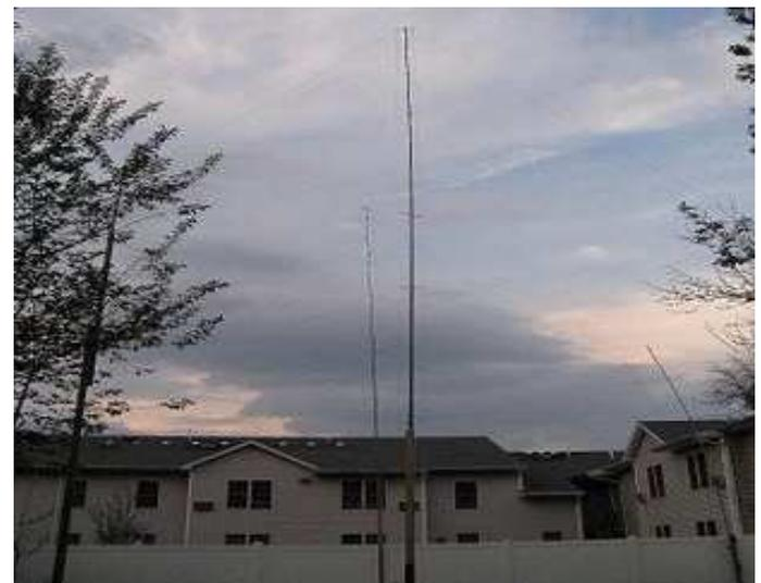
Long story short, a little pruning got me to 7.150 on both. I hooked up the previous phaselines to the outside corners and checked at the radio. I got a 1.7 swr in each direction, workable with no tuner required.
