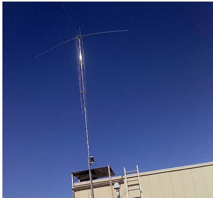
The weather was nice and not too windy for the work. While Bob and Ross ran coax between penthouse #6 and #4 using some Dacron line, the rest assembled the various antenna sections together as well as assembling the counterpoise system cables. Some of the grounding lugs had to be replaced as the supplied ones had no chance of fitting around a 1/4" bolt. Also, we had to solder the cable used for the counterpoise.
