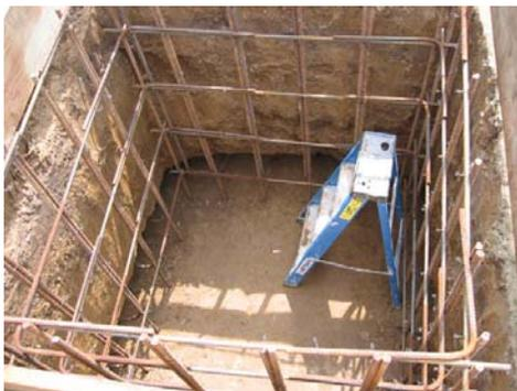
A big hole in the ground for a 64' tower. Note the bell shape flare at the bottom.
